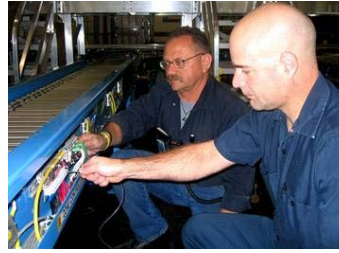
Denver PDC Electronic Technicians Luis Vasquez, left, and Mike Sharpe re-wire the flat sorting machine automated tray conveyance system.
