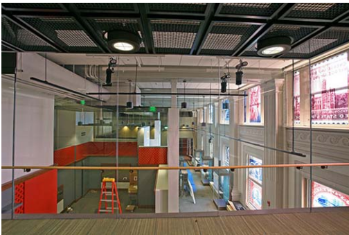
Interior Pic of Gallery Under Construction
